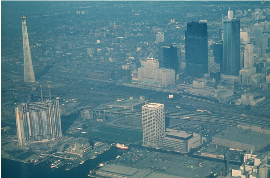
The newly-built Toronto Star building ca. 1974, with the under-construction CN Tower top left, and Ludwig Mies van der Rohe's Toronto-Dominion Centre top right. Source: City of Toronto Archives
