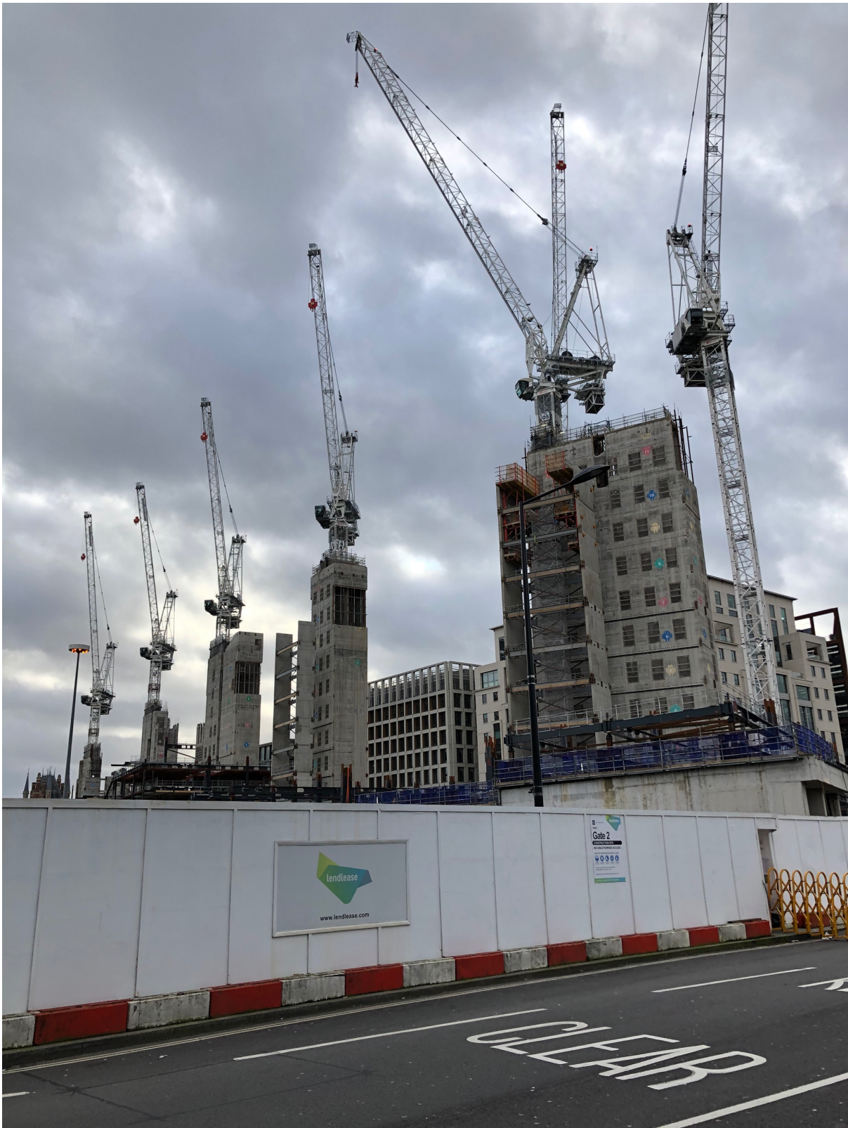
A parade of construction cranes indicate the scale of Google's 1,000 foot 'landscaper'. Source: Scott Rodgers
